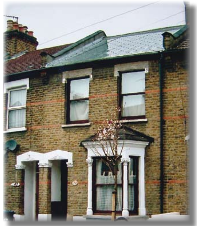
17m 2 for water heating
