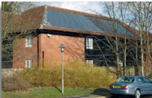
Hotel - 32m 2 for water pre-heating
