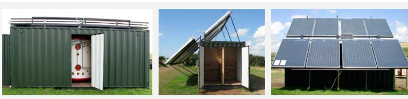
The standard cabin consists of 4 shower cubicles, 8 solar panels (24m<sup>2</sup>) on two roof mounted frames, with a 43w solar PV panel supplying electricity for the unit. A central plant room contains a 3,000 litre heat storage tank, the solar pump and controls, and the wiring and plumbing.
