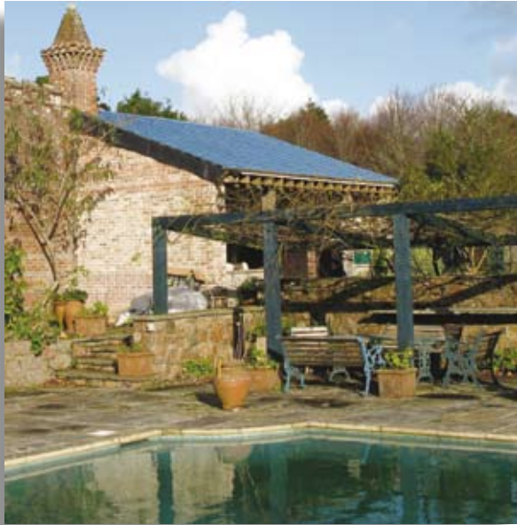
Jersey - 36m 2 of roof for pool heating
